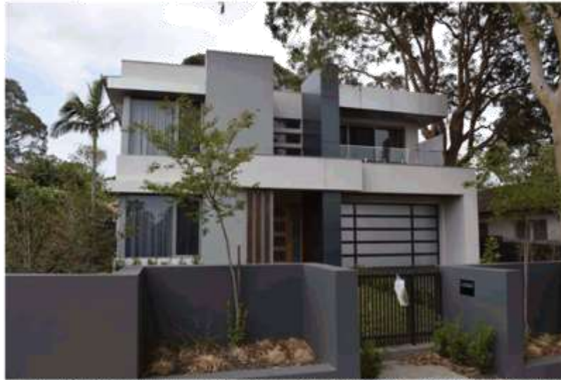
Photo 2 – Neighbouring property adjacent to subject site – 18 Arthur Street, Strathfield
