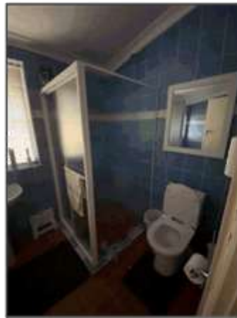
Figure 32. Internal view to existing bathroom.
