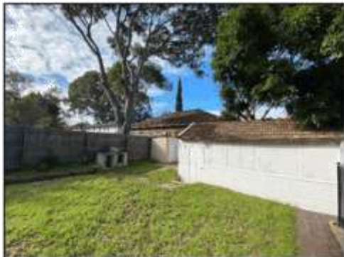
Figure 19. View to existing garage and metal shed within the rear yard of the subject site, facing east.
