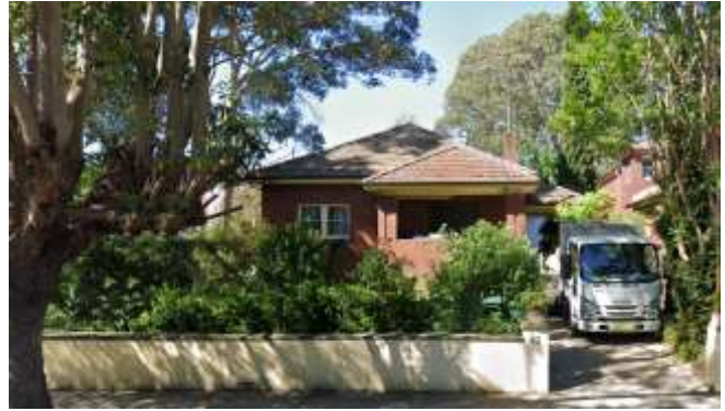
Image 4: 42 Bates Street (adjoining the rear)
