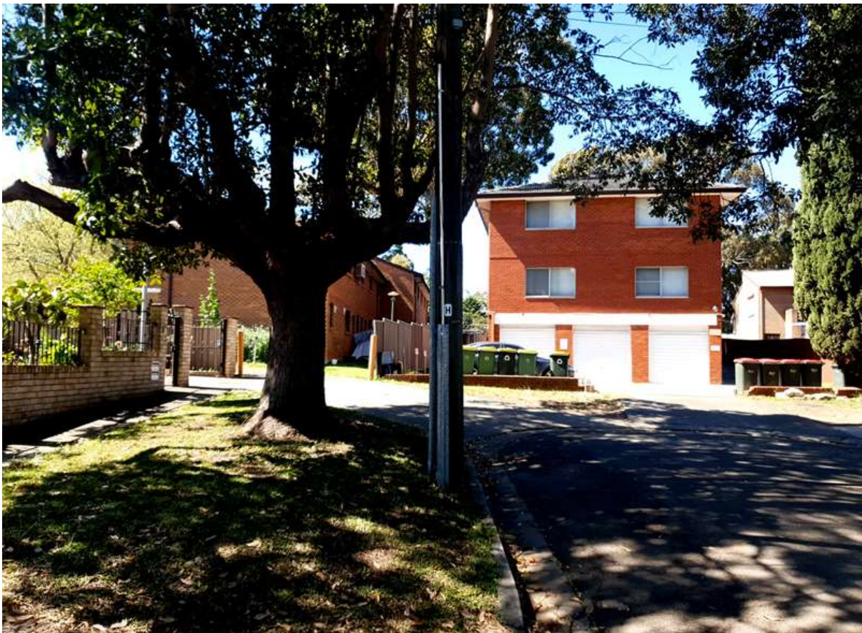
Figure 10. Image showing the residential flat building at the end Gees Avenue.
