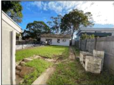
Figure 17. View to the rear (south-eastern) elevation of the original dwelling as viewed from the rear yard of the subject facing north.
