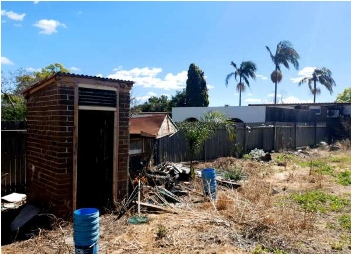
Figure 7. Outbuilding located at the rear of the site.
