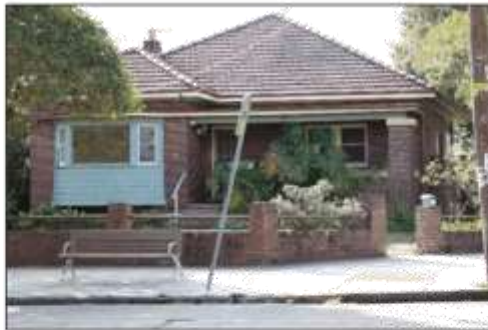
Figure 2: 51 Barker Road as viewed from the street.
