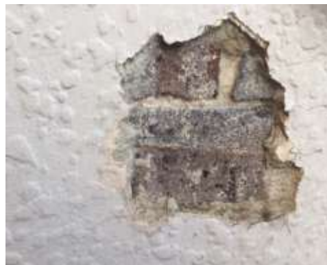
Image 16: Thick render has been chipped away to show stone work below.
