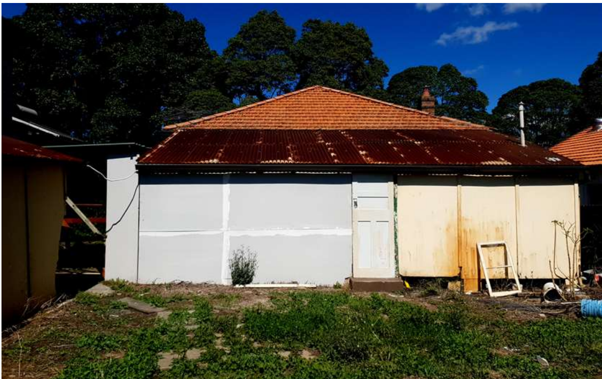
Figure 8. Rear elevation of the existing dwelling house on the site.
