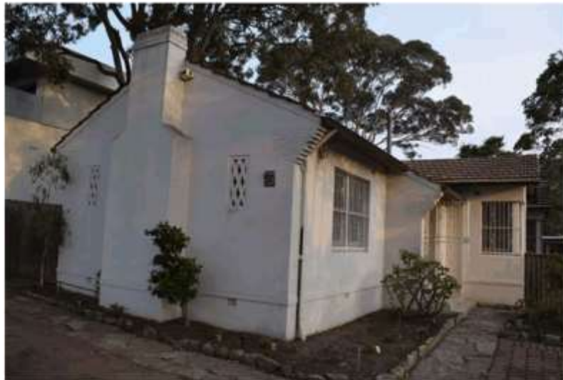
Photo 1 – Subject Site – 20 Arthur Street, Strathfield
