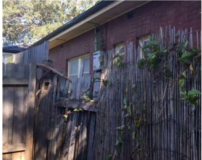
Image 18: Corner of yard adjoining Bates Street.
