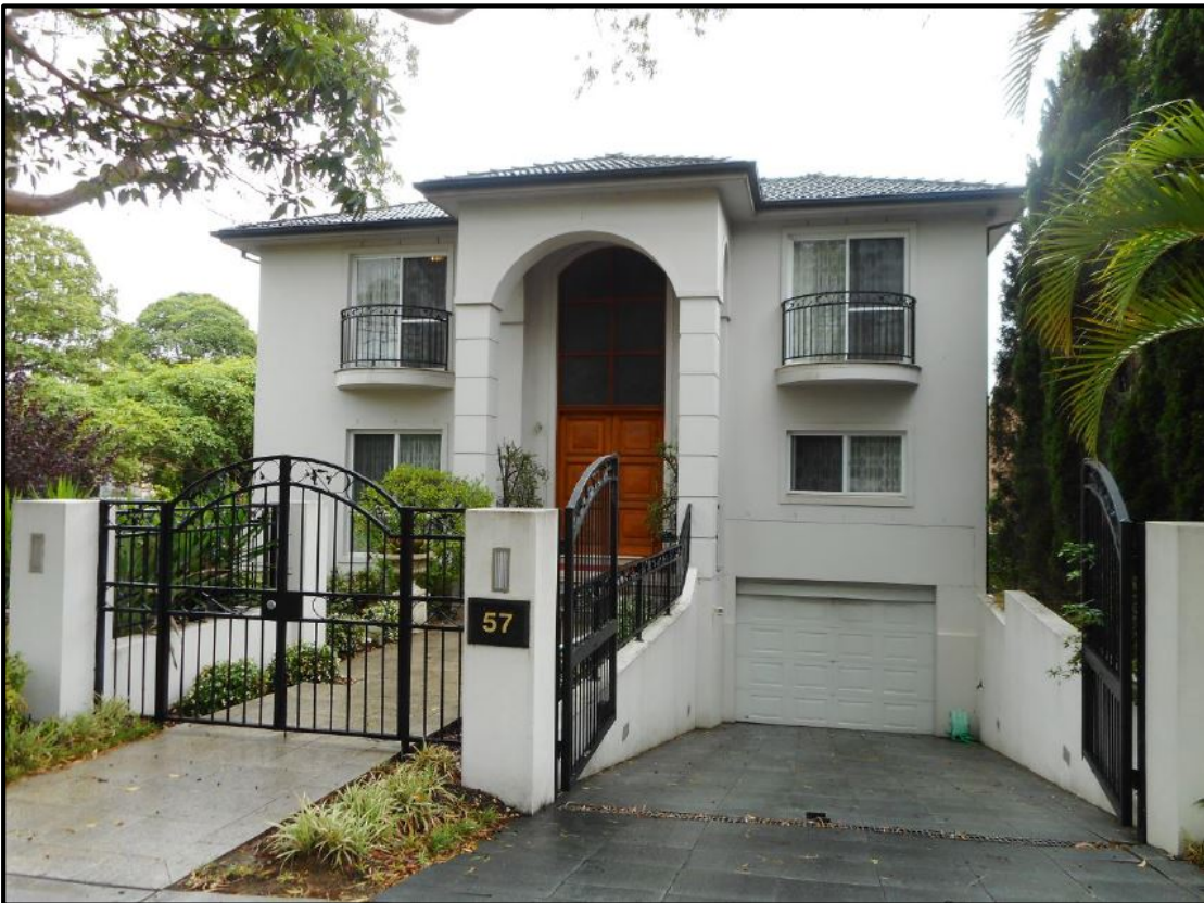
Figure 7: Existing dwelling house at No. 57 Oxford Road, Strathfield
