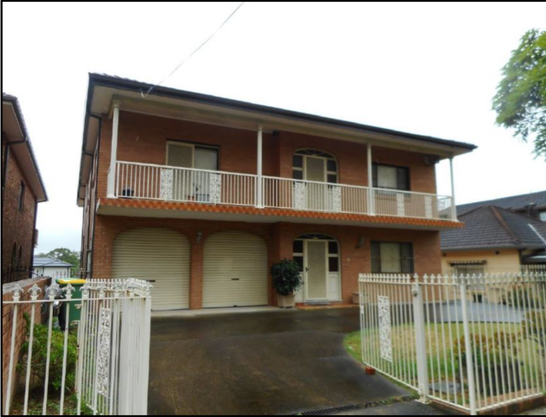
Figure 6: Existing dwelling house at No. 53 Oxford Road, Strathfield
