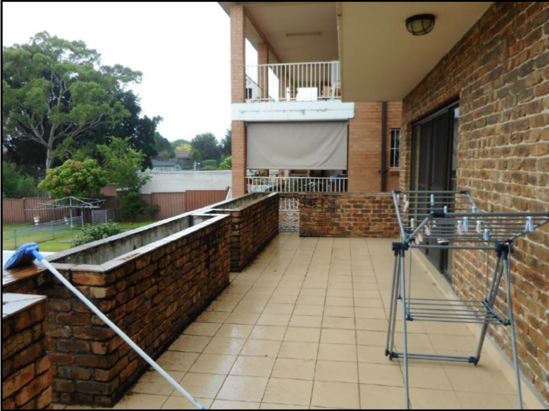
Figure 12: Existing ground floor balconies within the subject site and No. 53 Oxford Road, Strathfield
