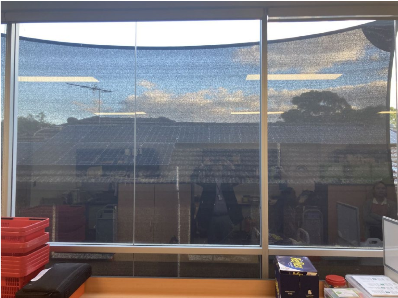
Figure 13. First floor windows with the shade screen installed outside.
