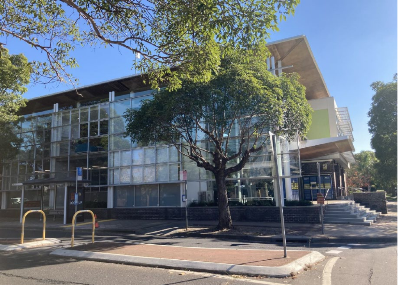
Figure 4. The eastern elevation of the library.
