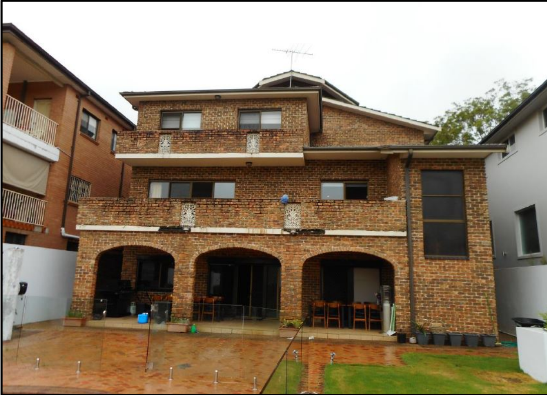
Figure 3: Rear of existing dwelling house within subject site
