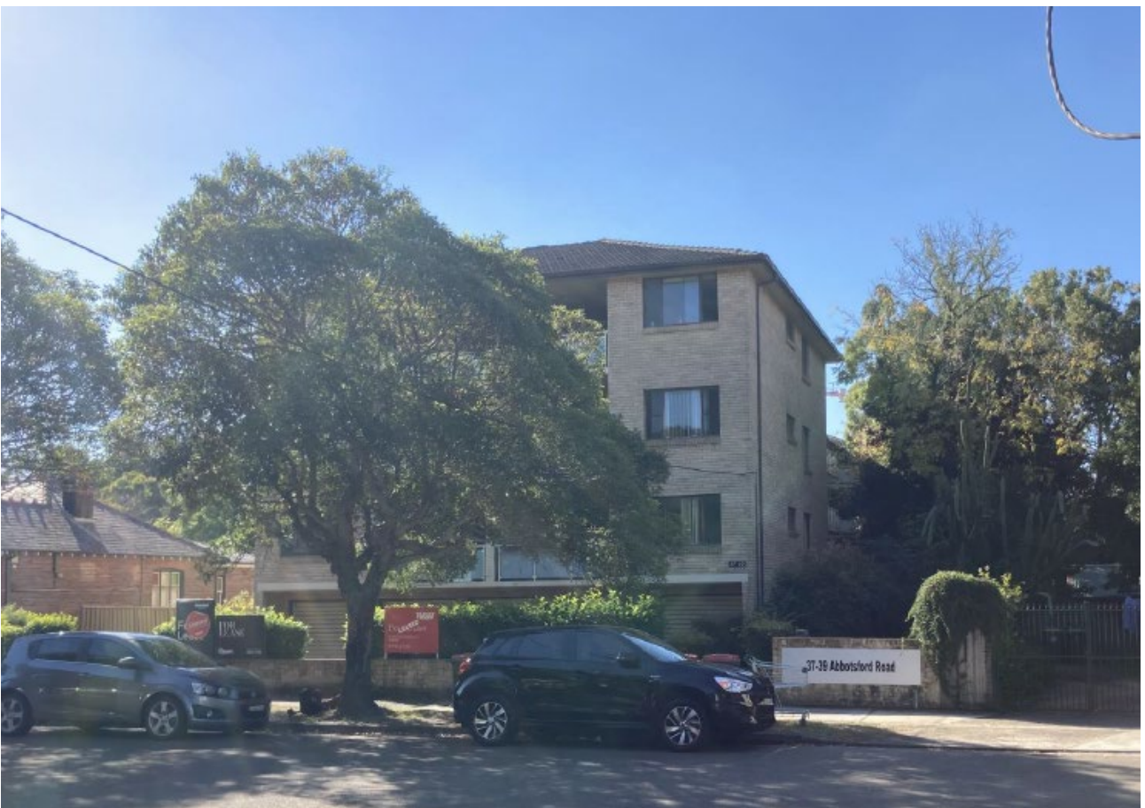
Figure 3. The residential flat building diagonally across from the library.
