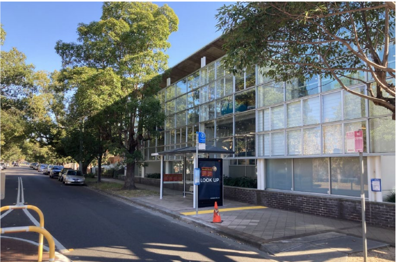
Figure 5. The eastern elevation of the library that is immediately adjacent to Rochester Street.
