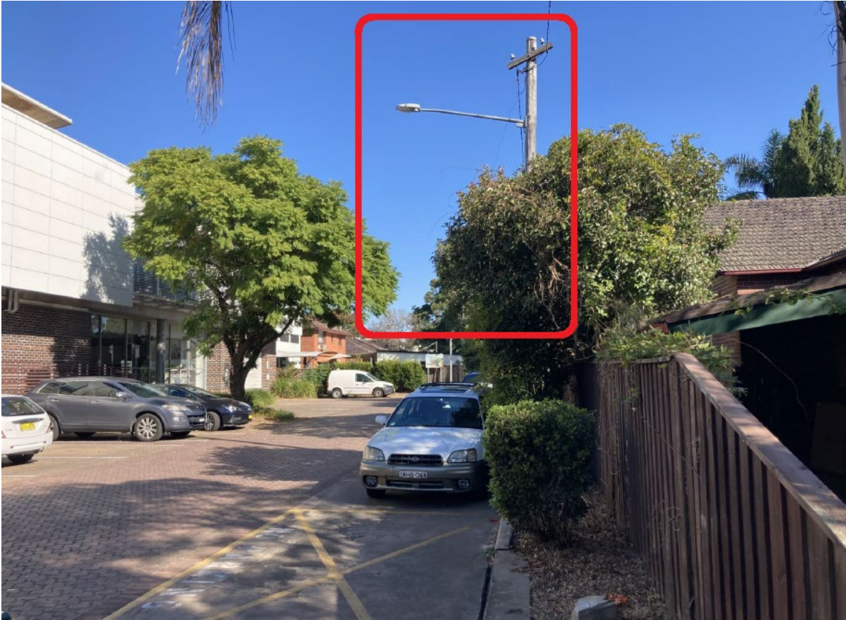
Figure 10. Image of the car parking area of the library with the existing lamp post outlined.
