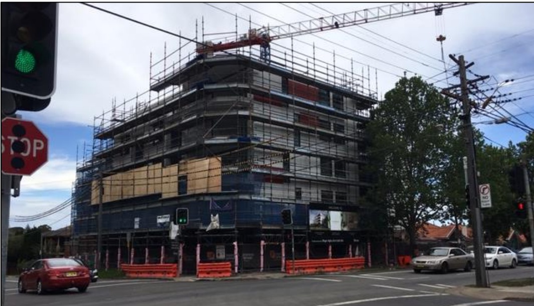
Figure 4 – View of 32-38 Underwood Road, Homebush (currently under construction)
