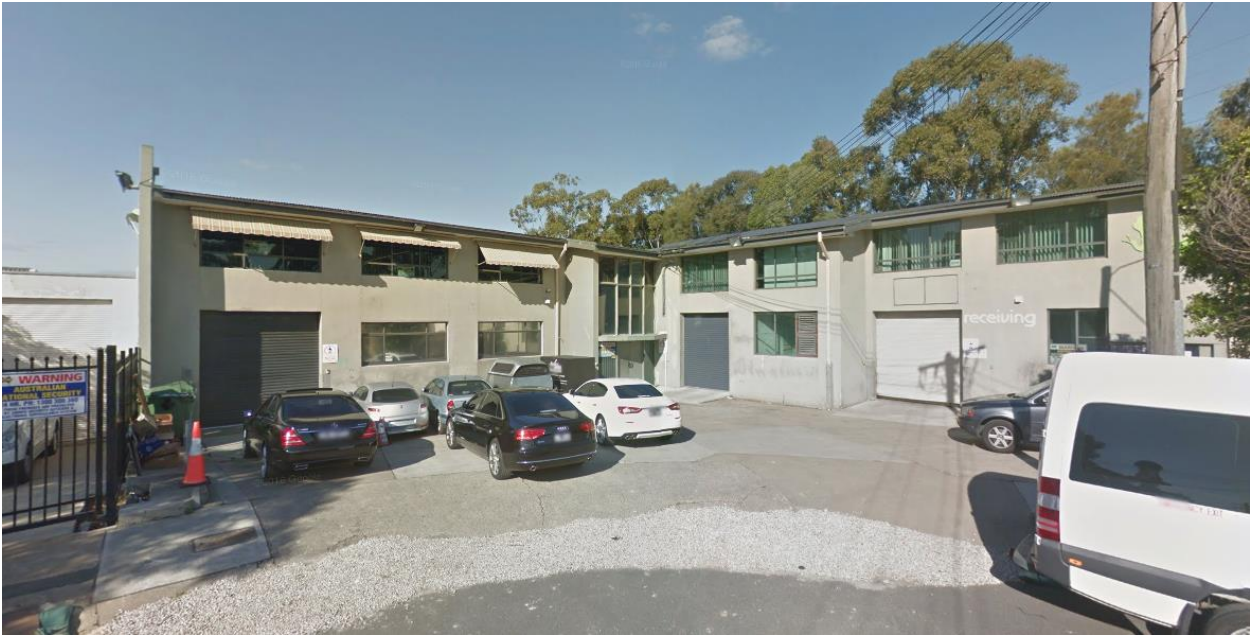
Figure 2: View of the existing premises from Dunlop Street (building on the left).
