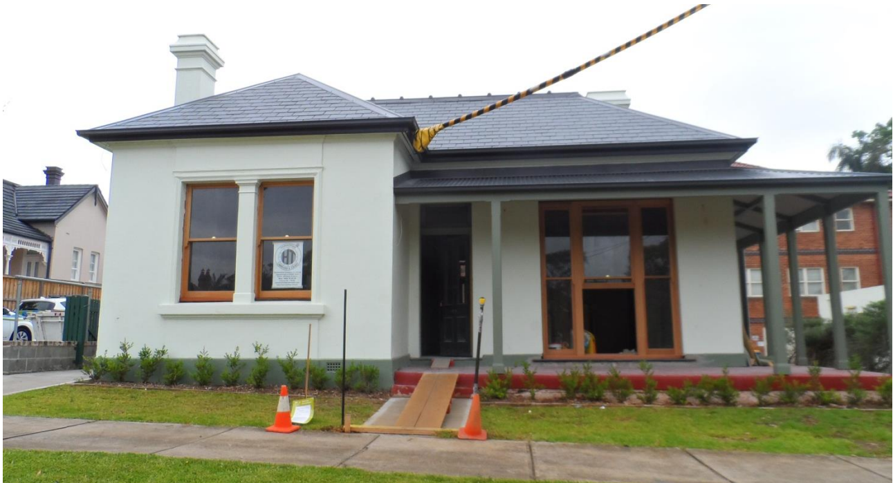
Figure 2: View of the existing dwelling from Redmyre Road.
