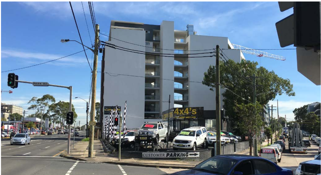
Figure 2: View of the No. 131 Parramatta Road, Homebush and No. 131A in the background.
