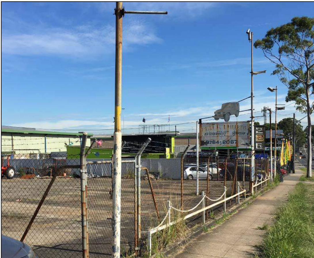
Figure 2: Existing Parramatta Road frontage of the subject site (looking west)
