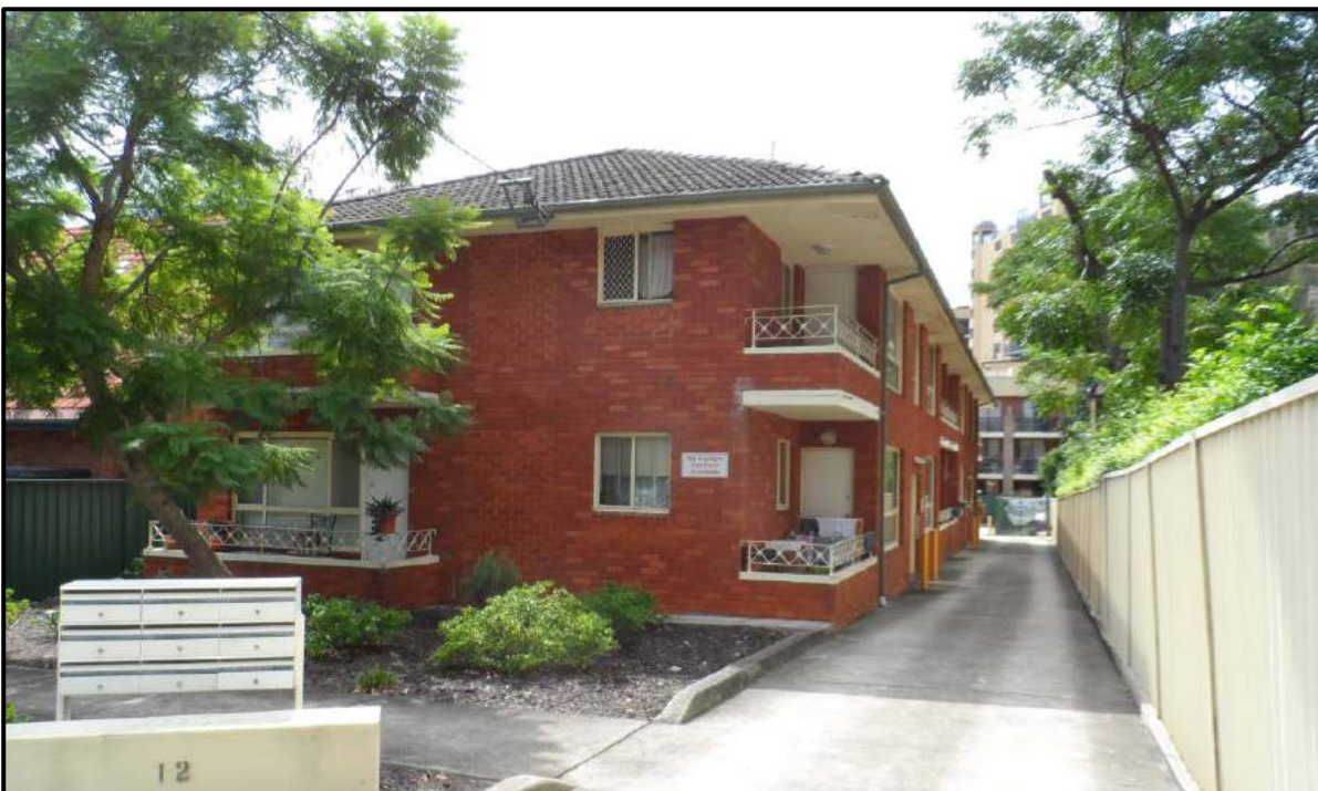
Figure 3: View of two (2) storey residential flat building at 12 Homebush Road, Strathfield.
