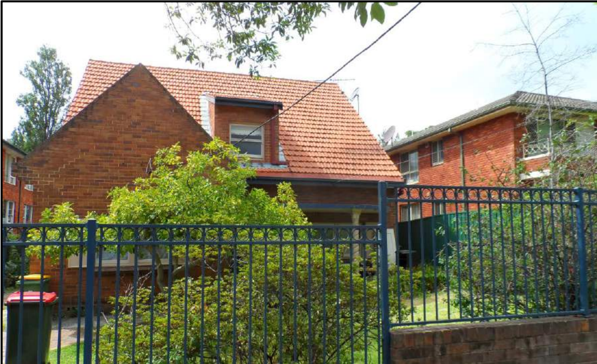
Figure 2: View of subject site.
