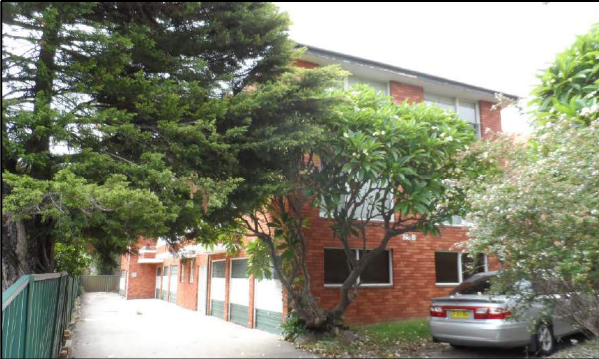
Figure 4: View of three (3) storey residential flat building at 8 Homebush Road, Strathfield.
