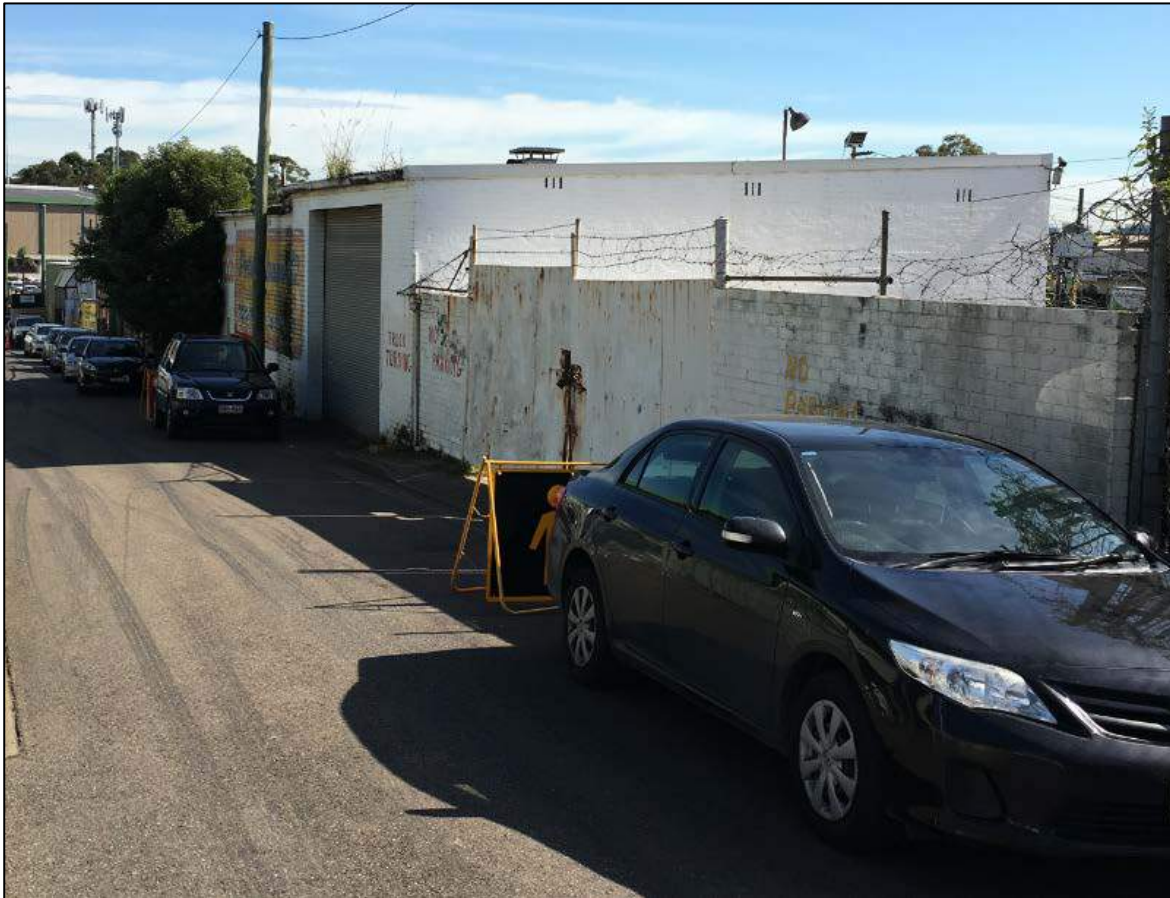
Figure 3: Existing Dalton Avenue frontage of the subject site (looking west)
