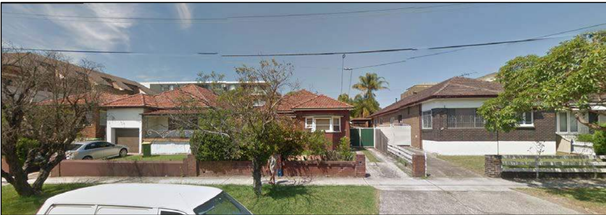
Figure 1: View of the four (4) existing dwelling houses at 22-28 Courallie Avenue.
