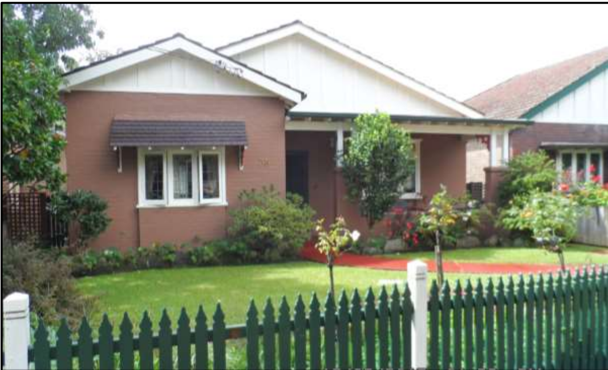
Figure 4: View of existing dwelling at 38 Loftus Crescent.
