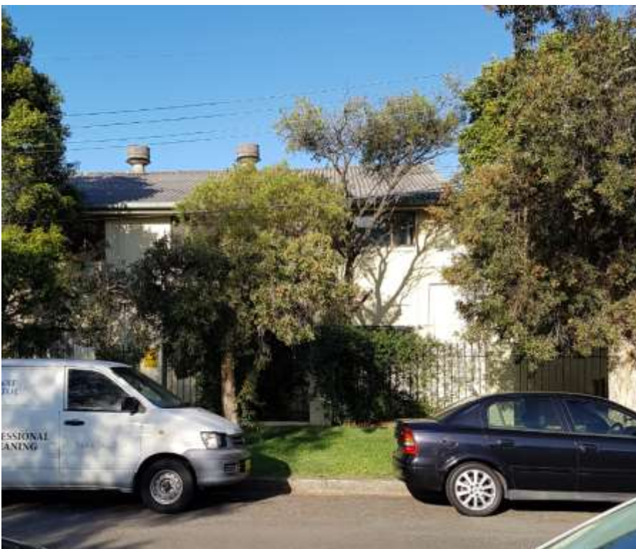
Figure 2: Existing development upon the subject site
