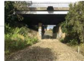
3. VIEW FROM SITE UNDER PUNCHBOWL ROAD
