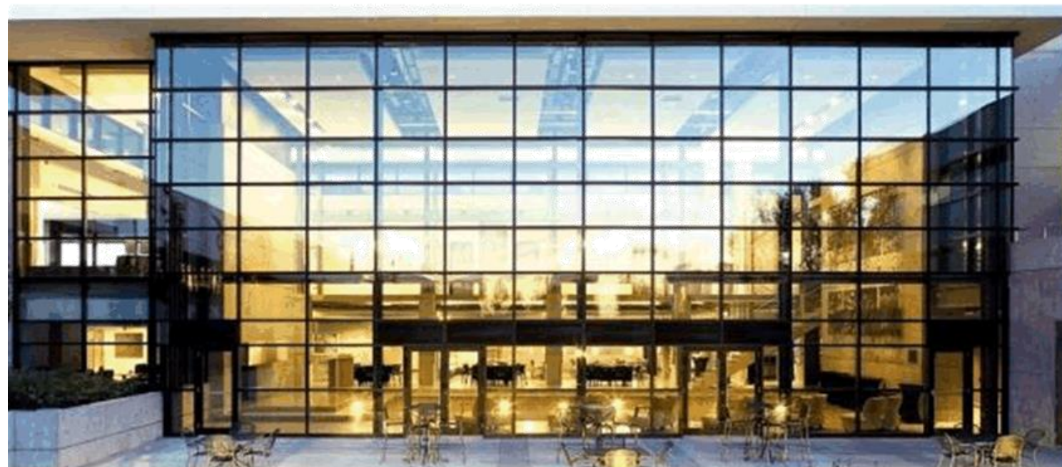
Full-height glass facade
