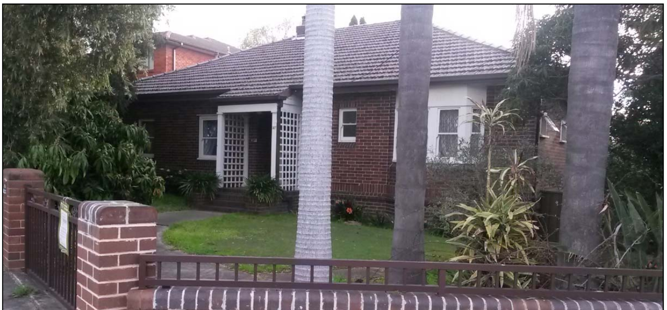
Figure 2: photograph of the existing dwelling at 387 Liverpool Road, Strathfield.
