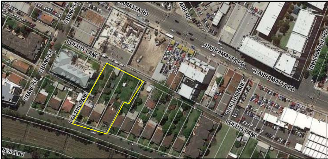
Figure 1: Aerial view of subject site and surrounding residential development.
