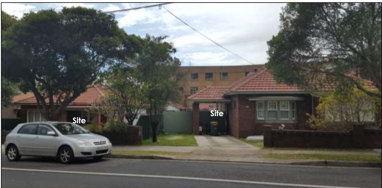
Figure 2: Site viewed from Water Street
