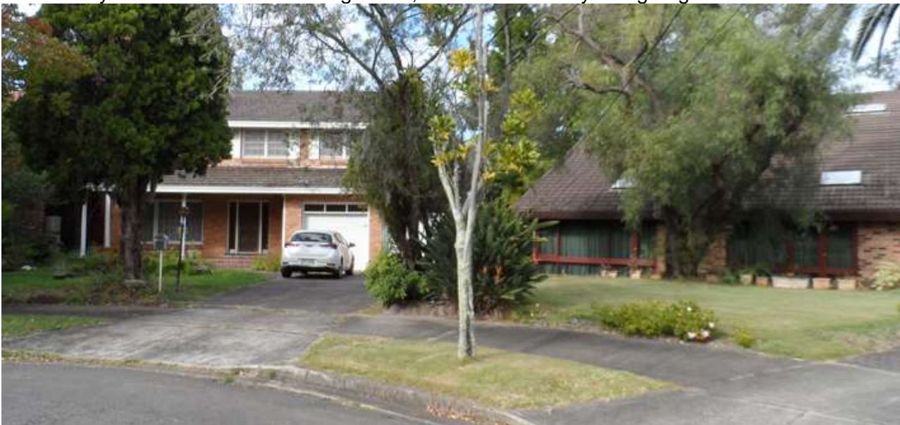
Figure 5: View of existing dwellings at No. 5 and 6 Summit Place.
