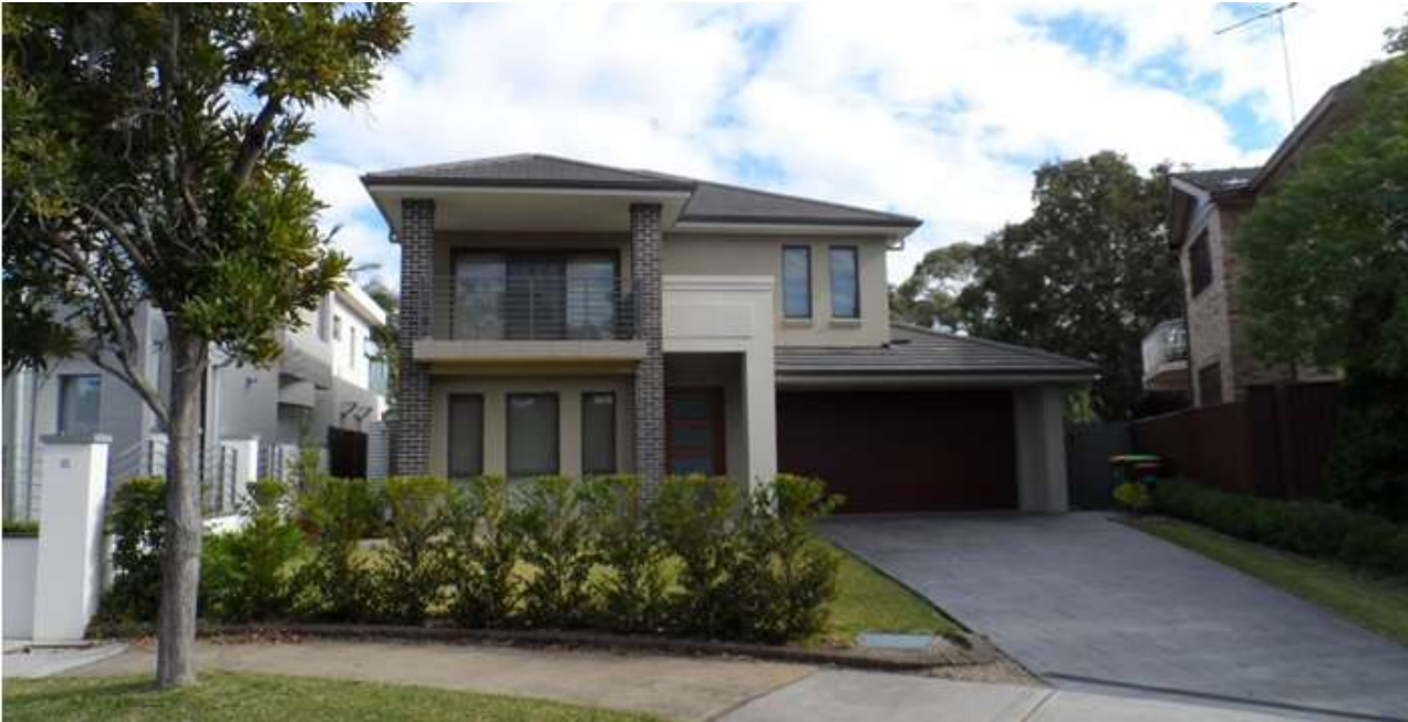
Figure 4: View of existing dwelling at No. 9 Summit Place.
