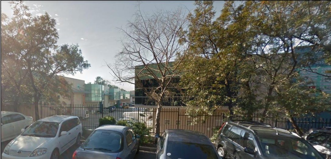
Figure 5: Easterly view of the existing industrial warehouses at 6-20 Braidwood Street, Strathfield South.
