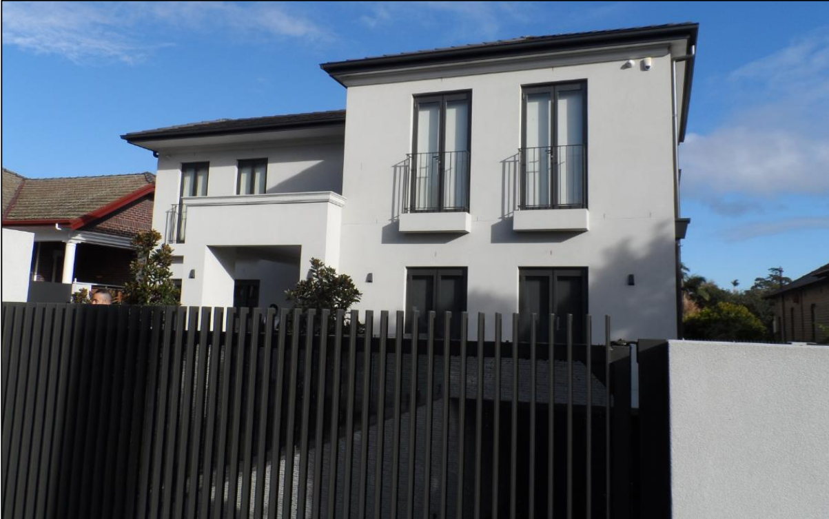
Figure 2: Westerly view of the subject site from Homebush Road.
