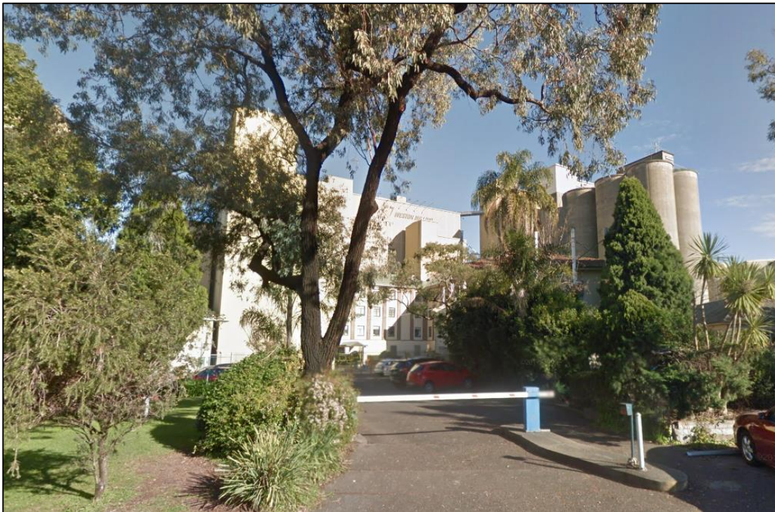
Figure 4: Westerly view of the driveway to the subject site (George Western Foods Feed Mill) from Braidwood Street.
