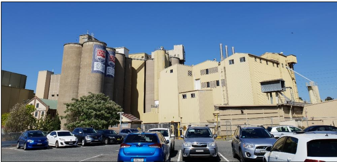
Figure 3: Westerly view of the subject site (George Western Foods Feed Mill) from private car park.
