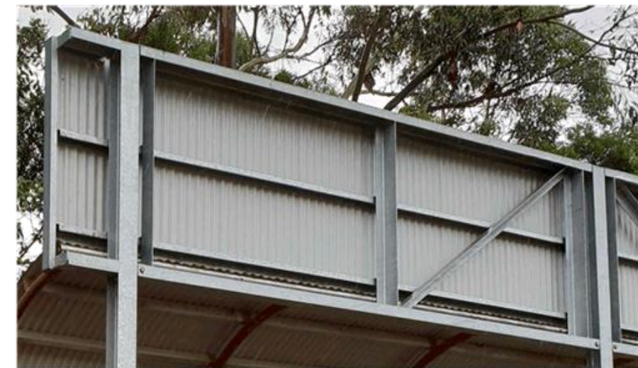
Figure 1 - Existing wall illustrating the final construction goals
