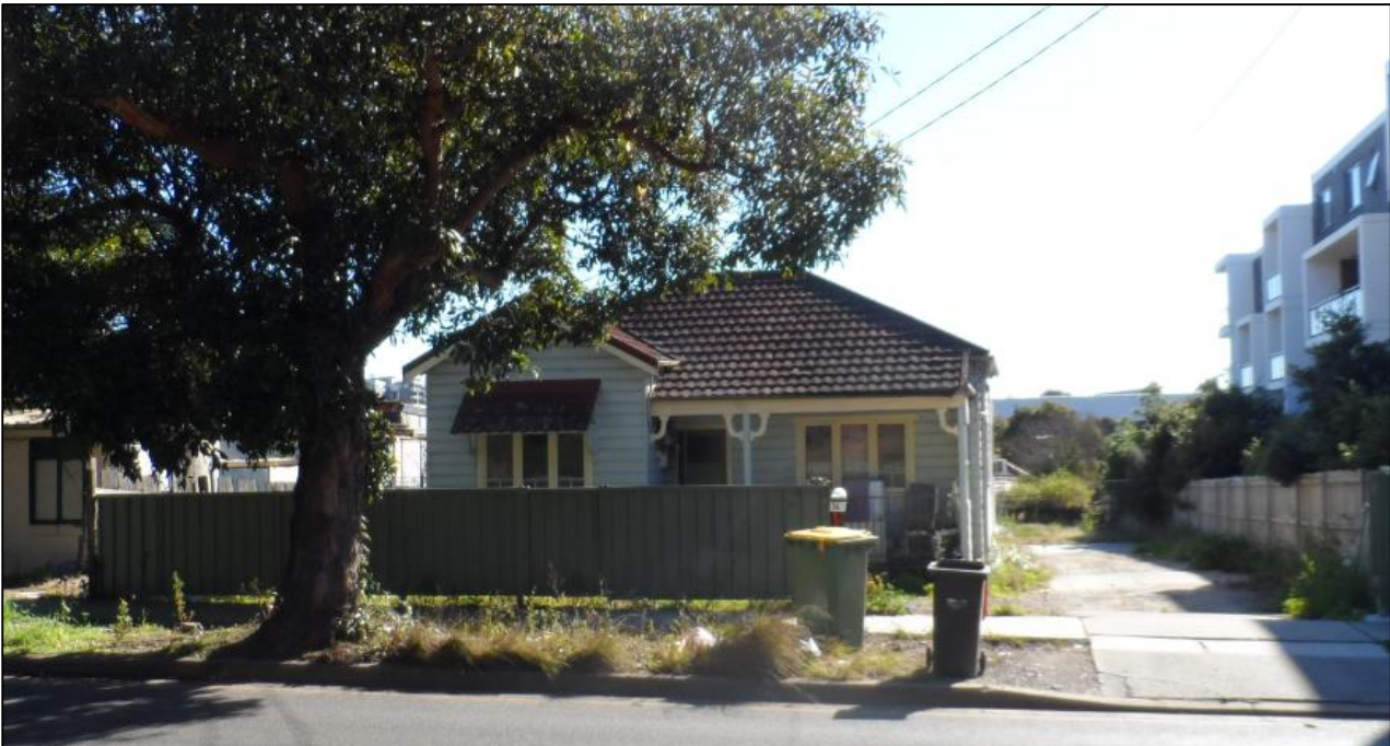
Figure 2: View of the subject site from Marlborough Road.
