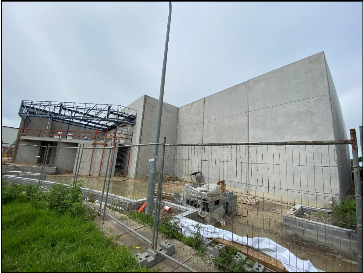
Figure 2: The approved warehouse development within the subject site and under construction.
