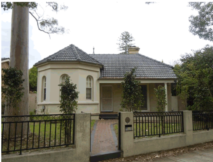
View of No. 44 Redmyre Road, Strathfield (Source: The Author, November 2017)
