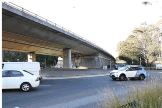
Figure 8 Homebush Bay Drive overpass, located immediately north of the site
