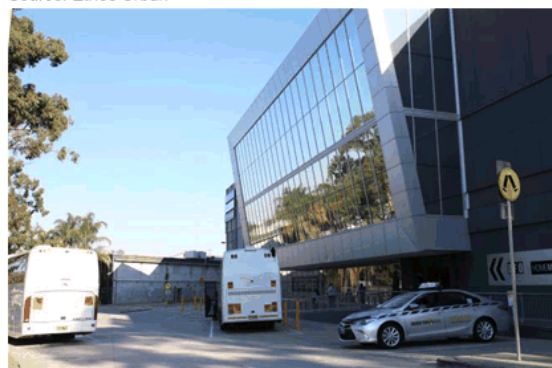
Figure 11 Coach parking located along the site's frontage to Underwood Road
