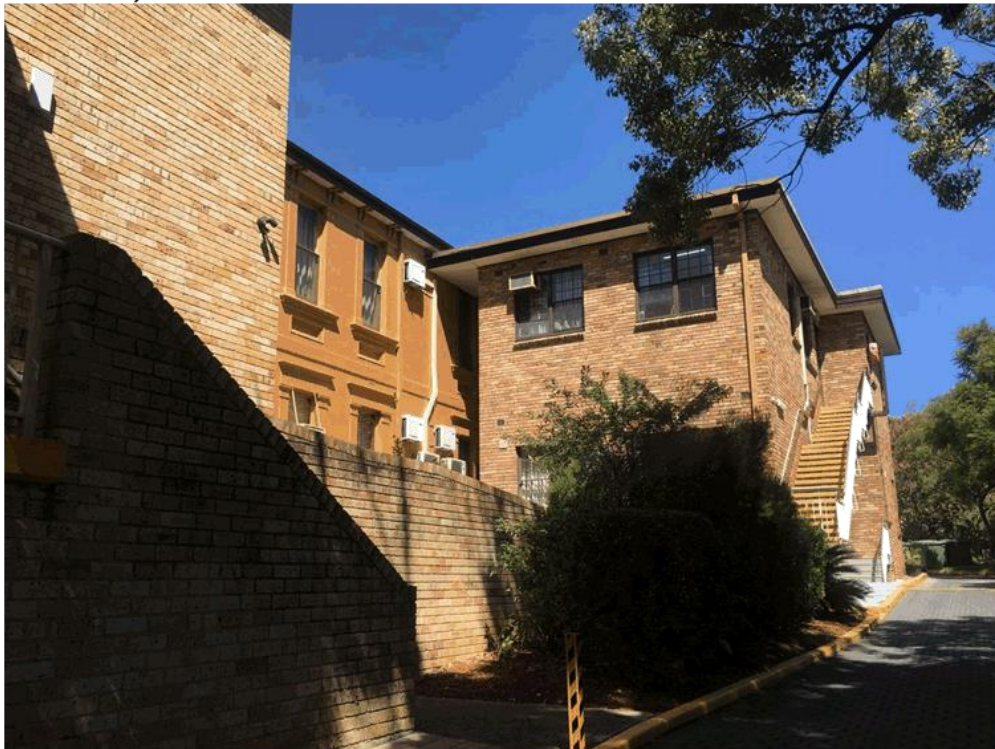
Figure 5: Portion of the south- western side elevation of the existing residential care facility
