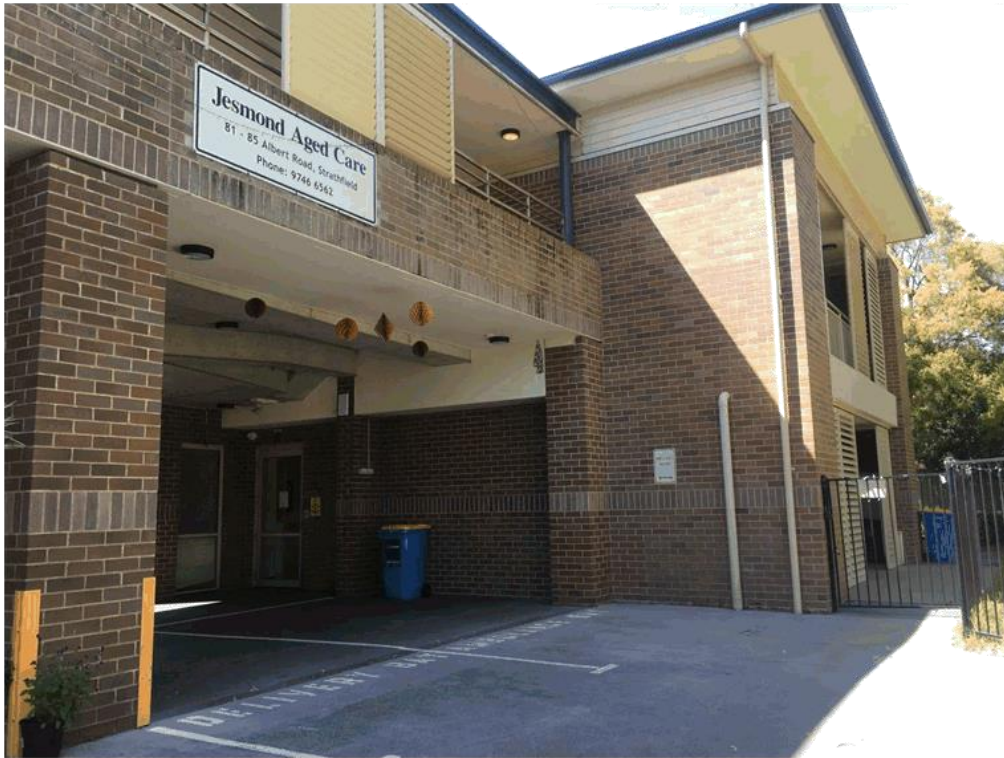
Figure 4: Portion of the front elevation of the existing residential care facility (orientated north- east)
