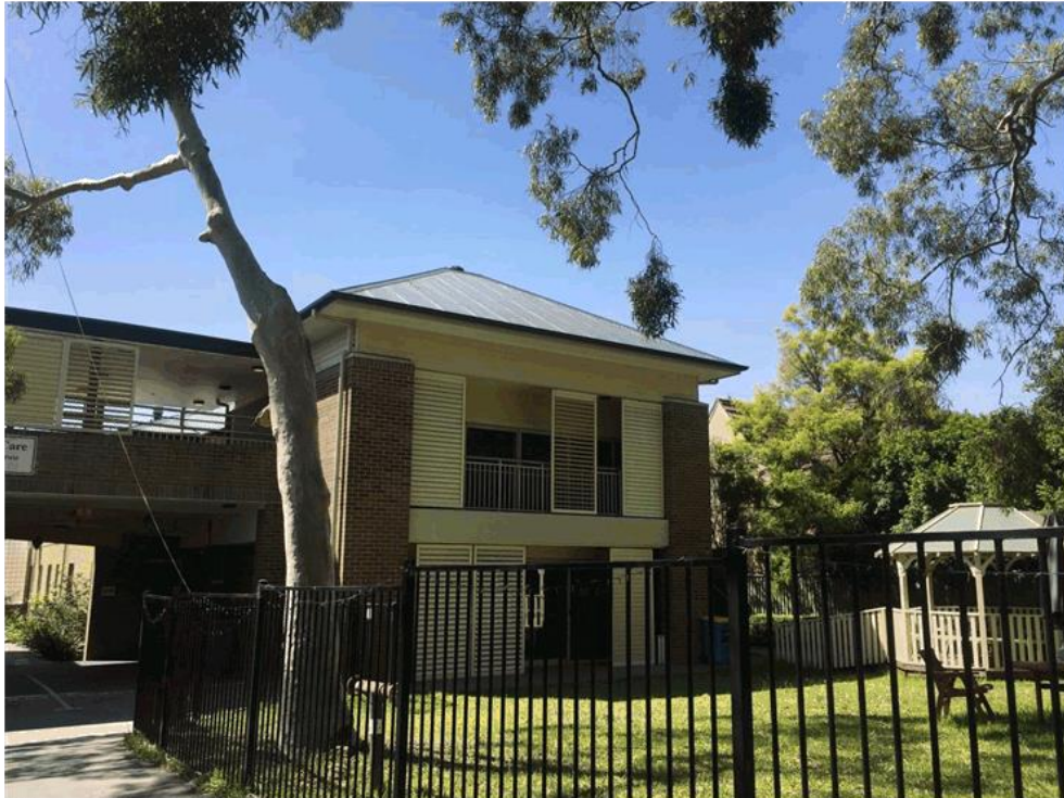
Figure 2: North- eastern portion of the front elevation of the existing residential care facility
