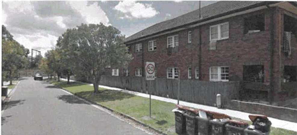
Figure 4: View north along Pilgrim Avenue
