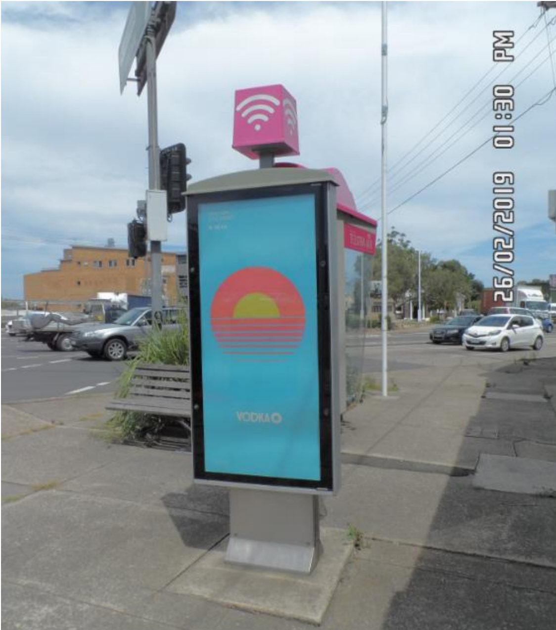
Figure 2: Existing payphone structure and associated signage.
