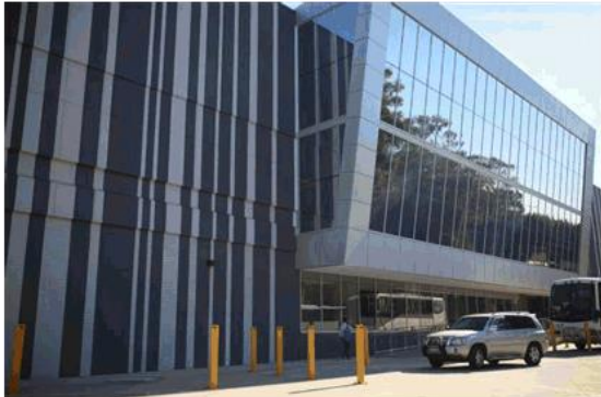
Figure 2 DFO Homebush's frontage to Underwood Road
