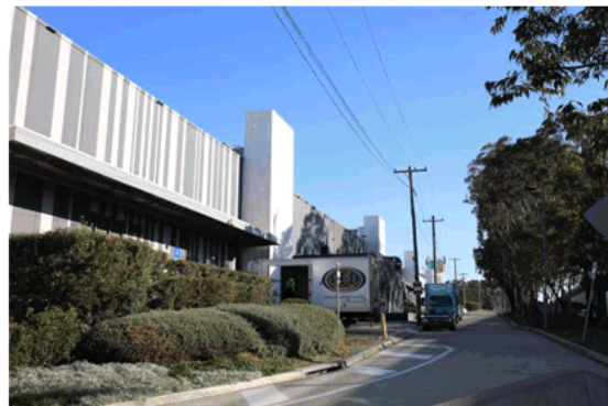
Figure 9 Loading entrance located adjacent Homebush Bay Drive (site's north-west boundary)
