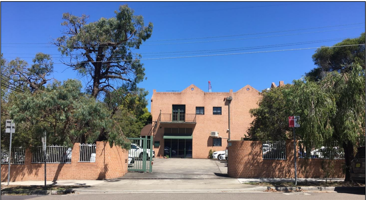
Figure 2: View of existing development from Pomeroy Street.
