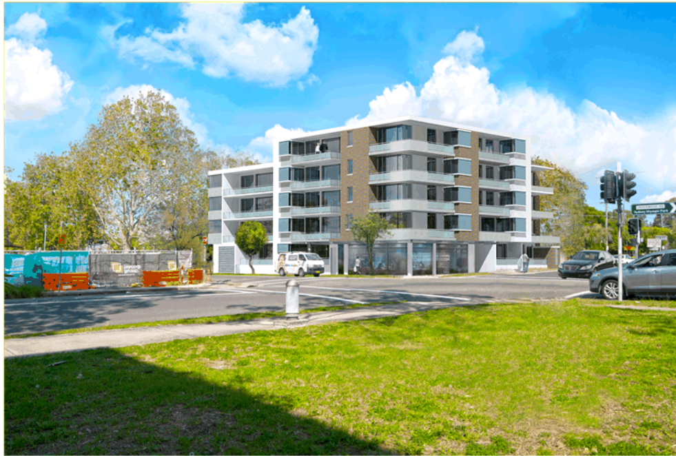
Figure 2 illustrating the design as amended and the landmark qualities of the building.
