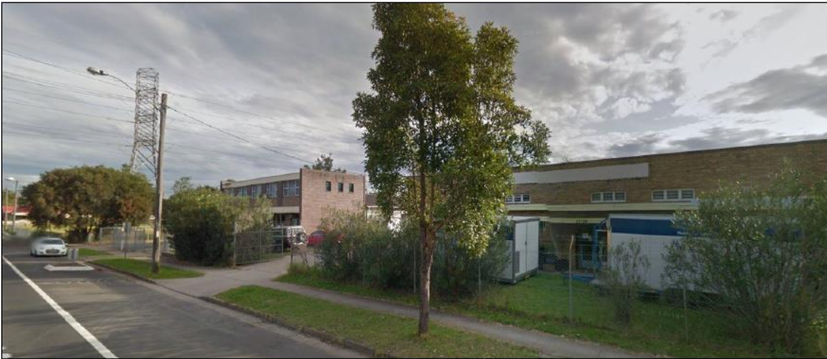
PICTURE 1 – PHOTO OF 25-33 WATER STREET
