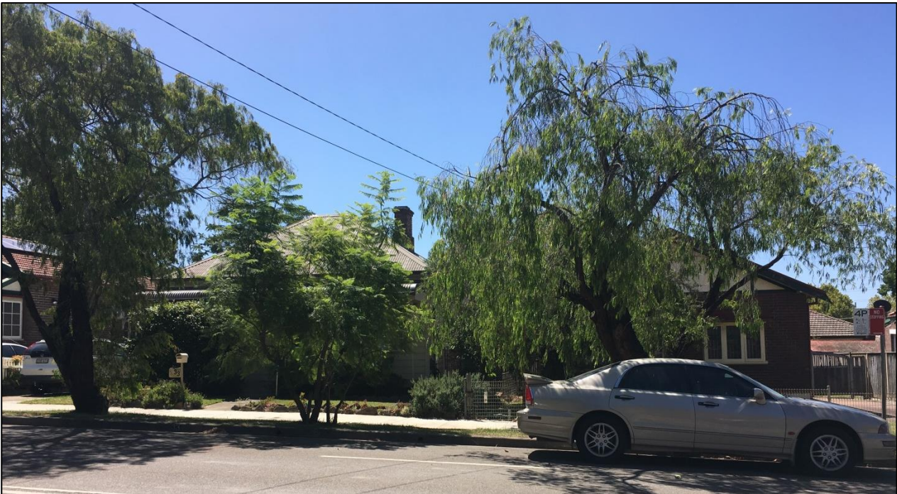
Figure 4: View of existing dwellings on Pomeroy Street.
