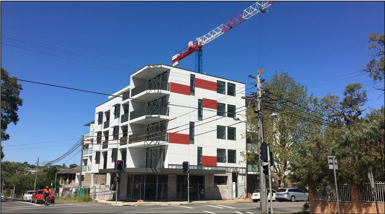
Figure 3: View of mixed use development under construction at 32-36 Underwood Road.
