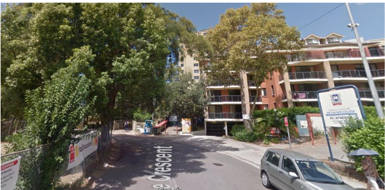
Figure 8. Cul-de-sac at the eastern end of The Crescent and eastern entry to the College.
