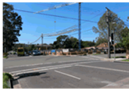
Photo 4 View of large Mixed-use development under construction opposite the site
