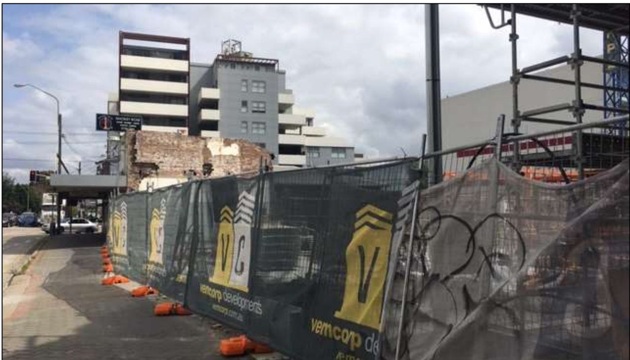
Figure 2: View of subject site. Construction of the site has commenced.
