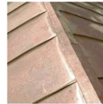
COPPER ROOF STANDING SEAM DETAIL PRE-PATINATED BRUSSETT COLOUR OR SIMILAR
