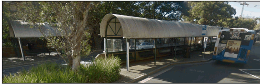
Photograph 2: Existing bus terminal opposite the Site.
