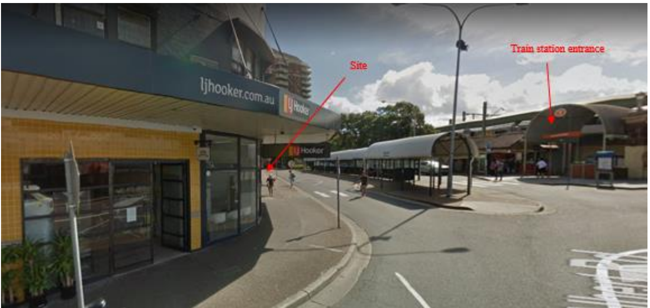
Figure 4. Western entrance to Strathfield Train Station, opposite the site.
