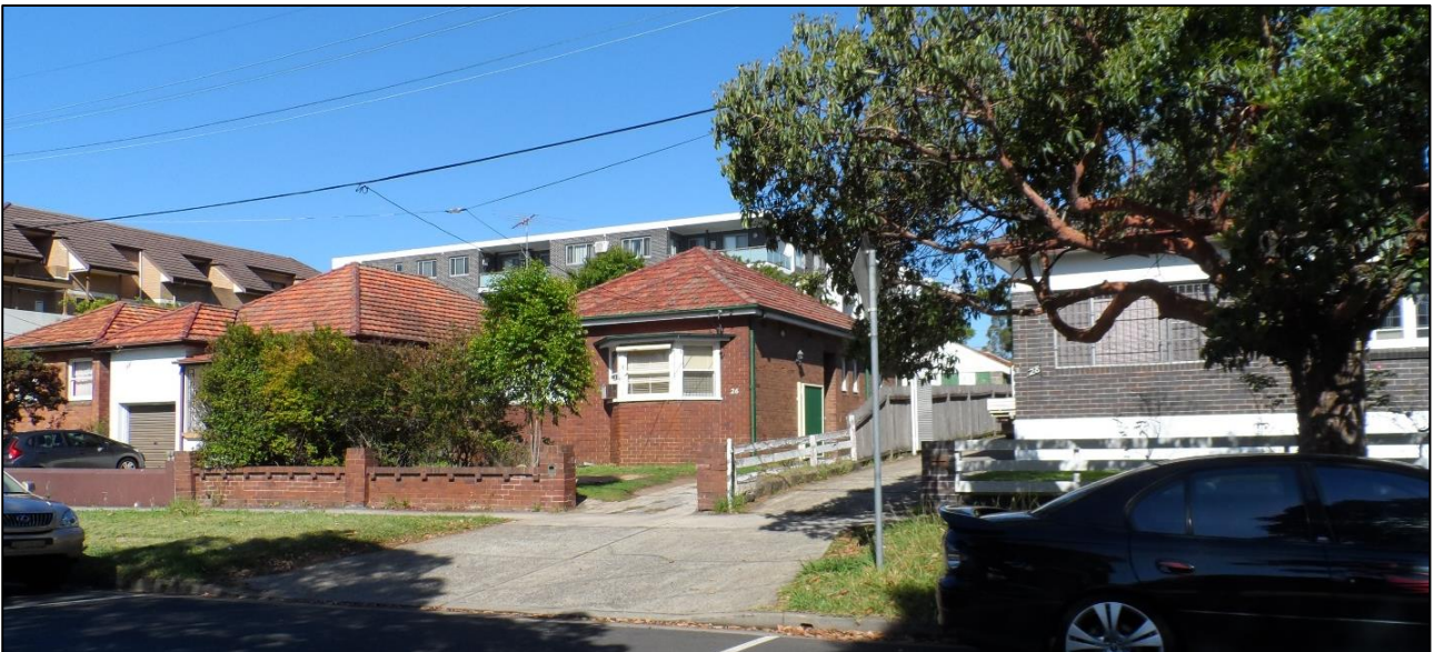
Figure 2: Existing dwellings at 22, 24, 26, and 28 Courallie Avenue.
