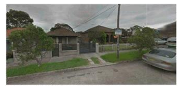
3. NEIGHBOURING BUILDING'S ON RIGHT OF PROPOSED SITE
