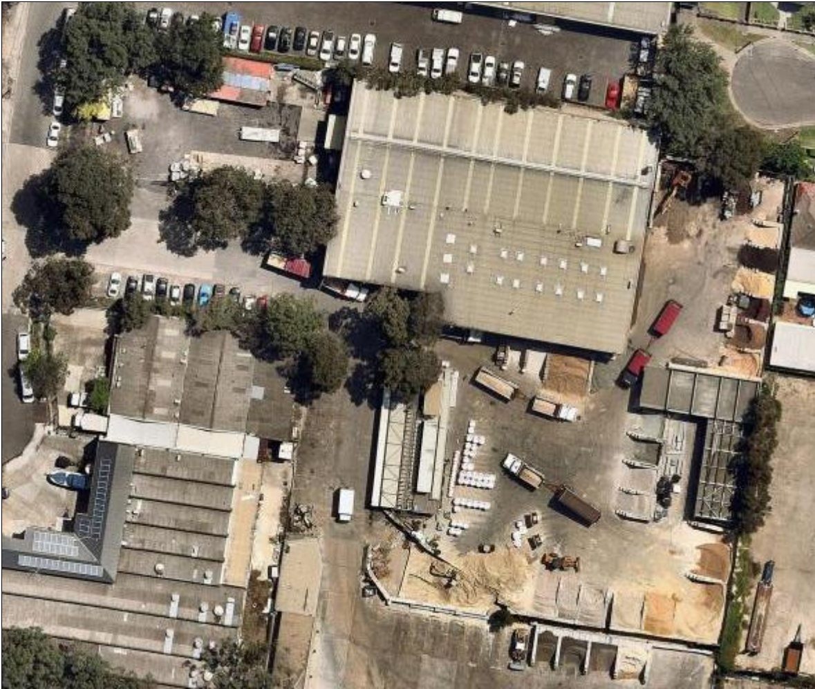
Figure 2: Aerial Photograph of Site (Builder's yard on right side of image)
