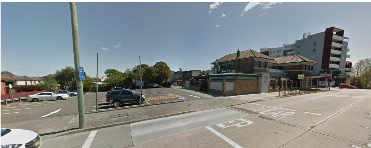
Figure 20. Existing 'Crossways Hotel' and ancillary at-grade car park to the north of the site on the corner of Homebush Road and Liverpool Road. The car park adjoins No. 247-249 Homebush Road (Figure 19).
