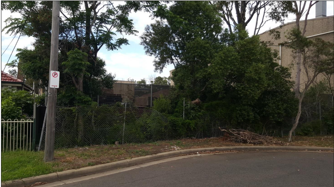
Figure 8: Southerly view of the interface between the site and adjoining dwelling house and William Street
