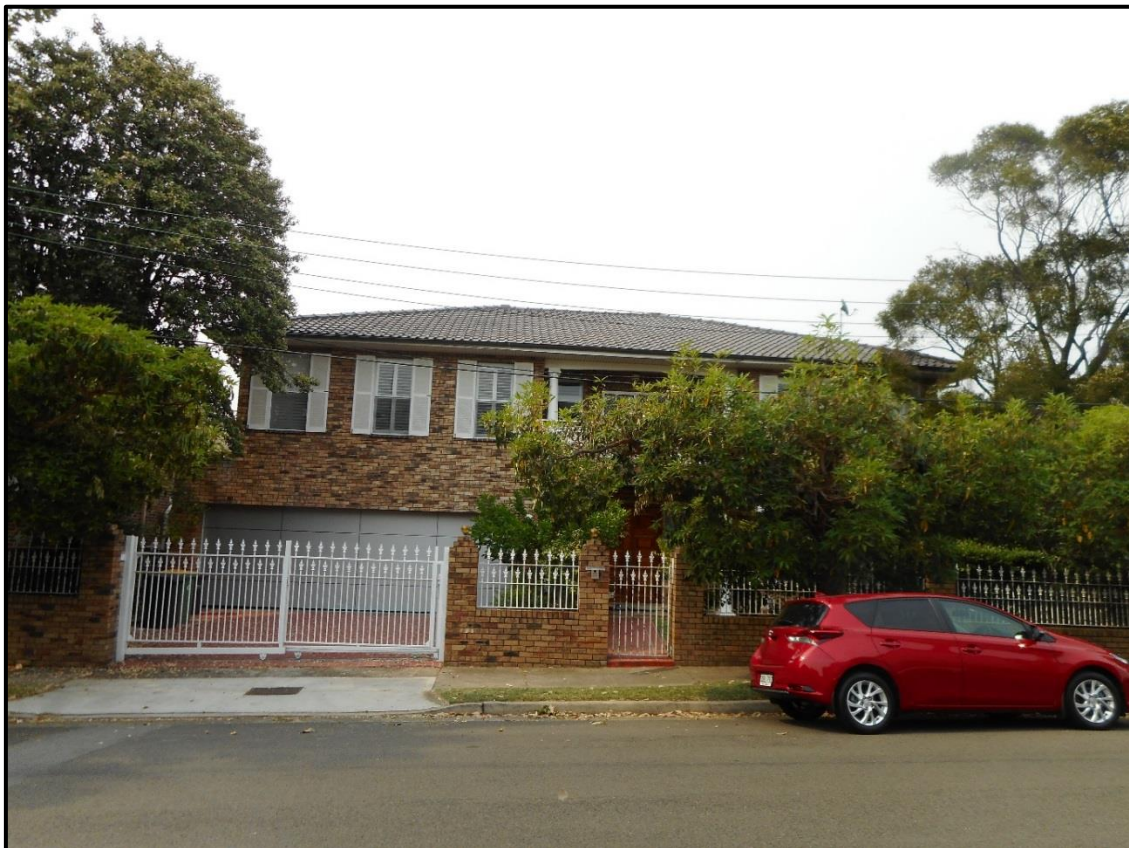
Figure 7: Two (2) storey residence at No. 18 Highgate Street.
