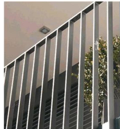
F - METAL BALUSTRADE | FENCE
