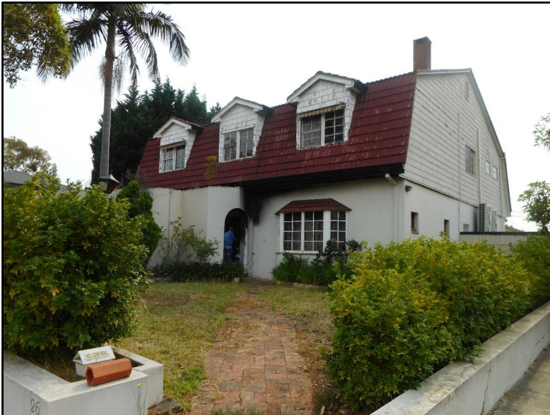
Figure 2: Front façade of existing dwelling featuring mansard roof and dormer windows.
