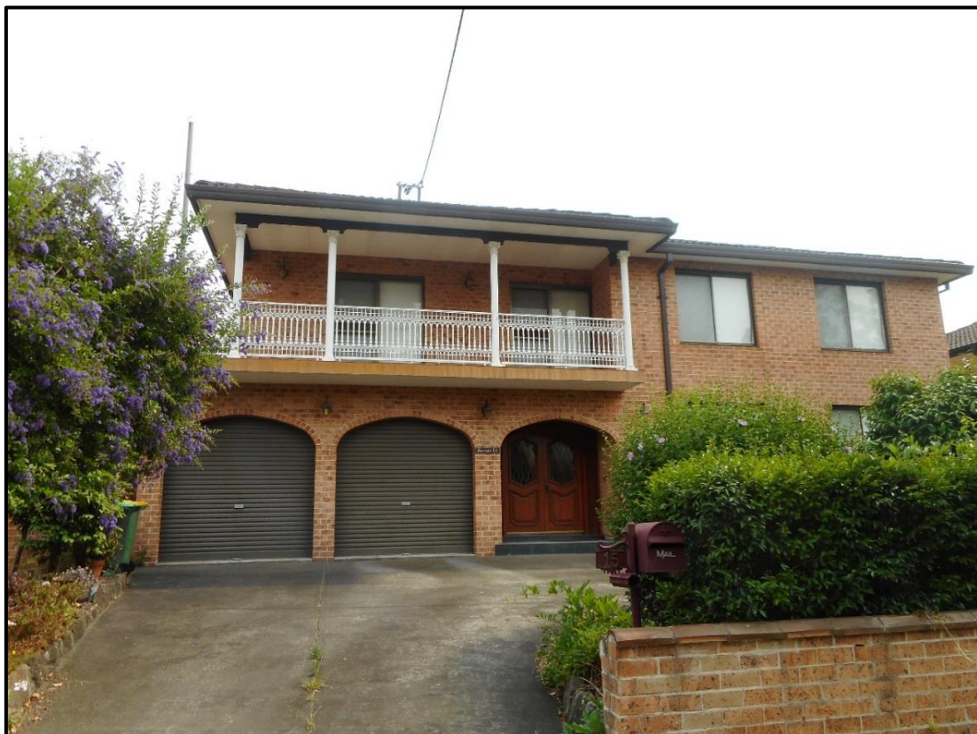
Figure 5: Two (2) storey residence at No. 15 Highgate Street.
