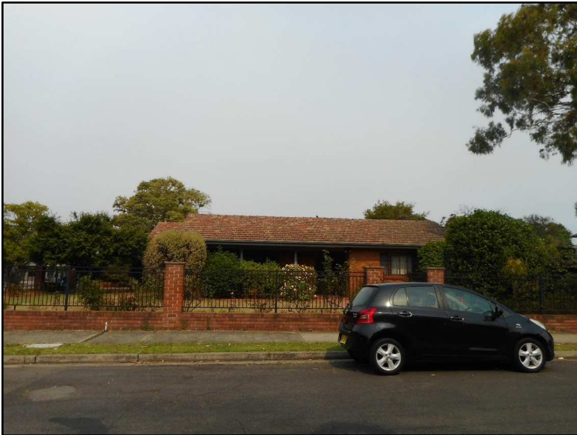
Figure 8: Single storey residence at No. 27A Kingsland Road.
