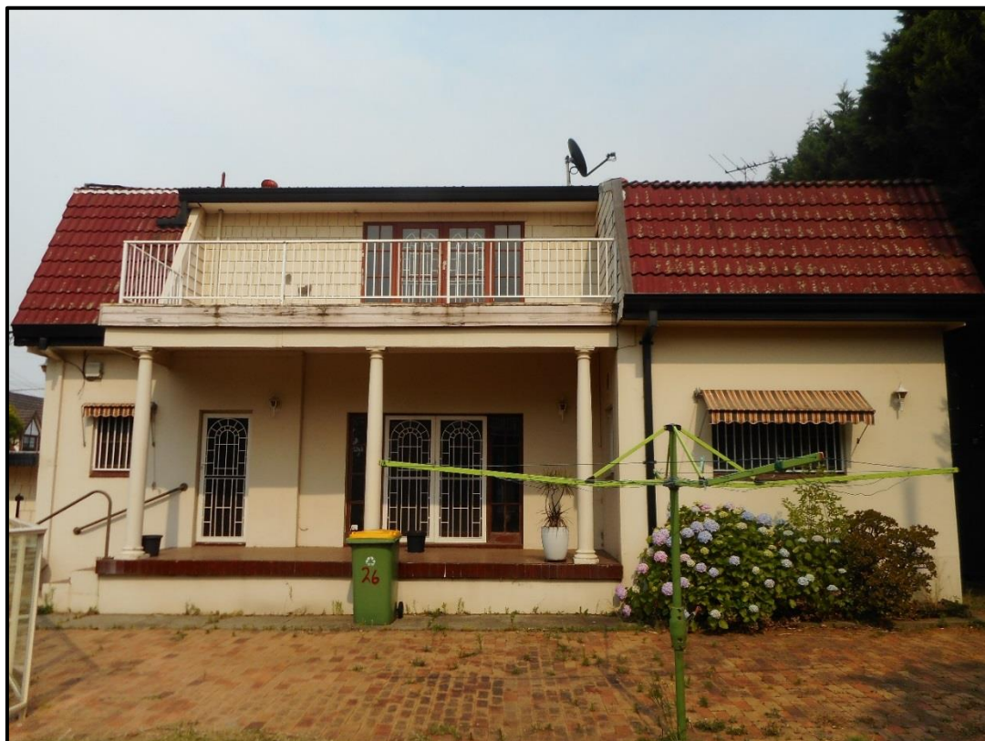
Figure 3: Rear (eastern) elevation of existing dwelling. Note the first floor balcony.
