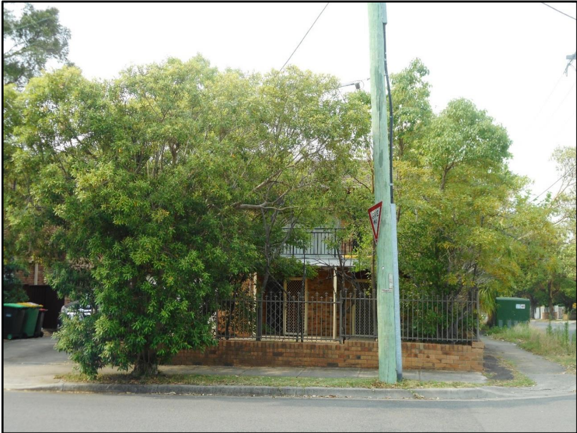
Figure 6: Two (2) storey residence at No. 20 Highgate Street.
