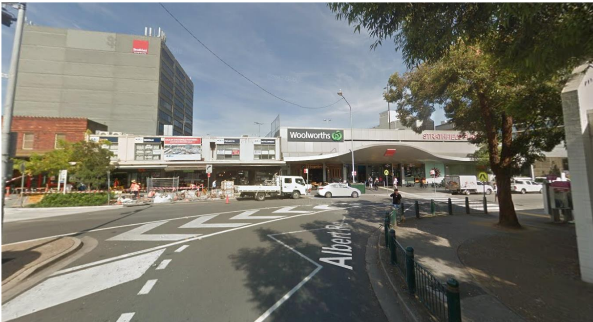
Figure 6. Churchill Avenue pedestrian entry to Strathfield Plaza looking south.
