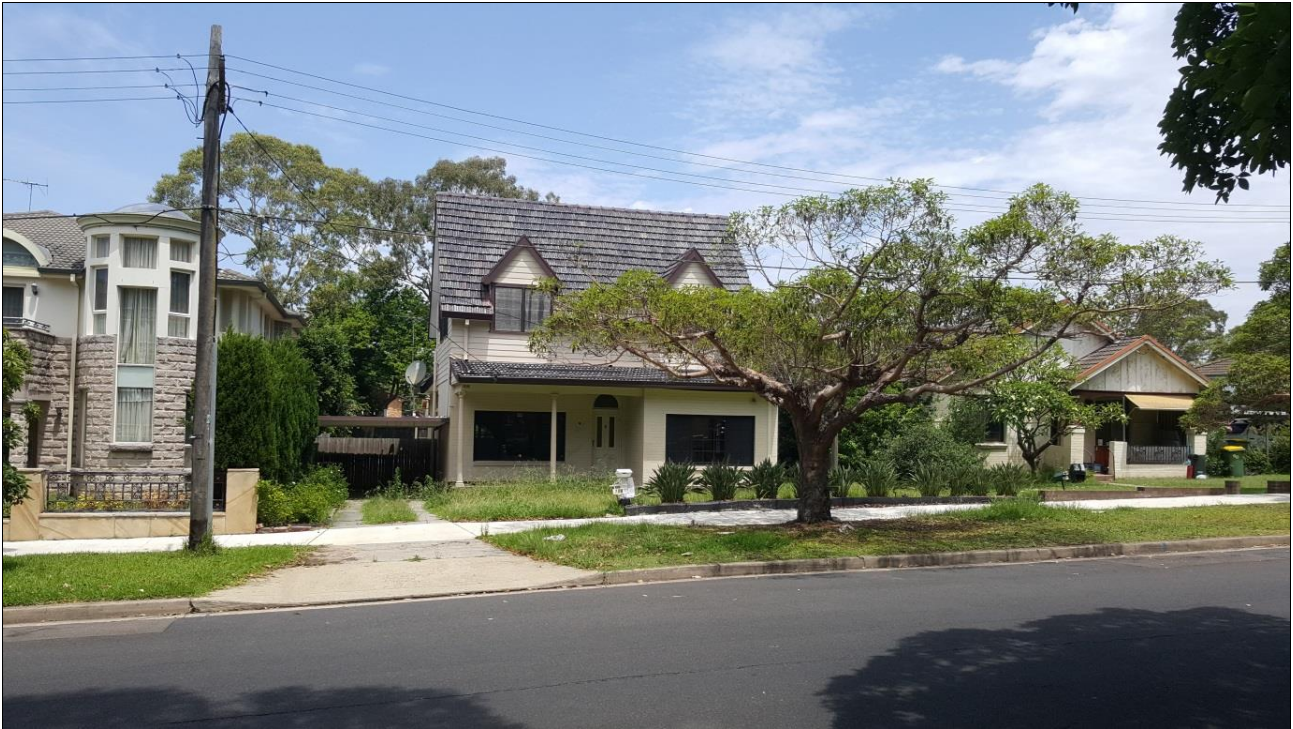
Figure 3: Southerly view of the site (at centre of image) from across the road
