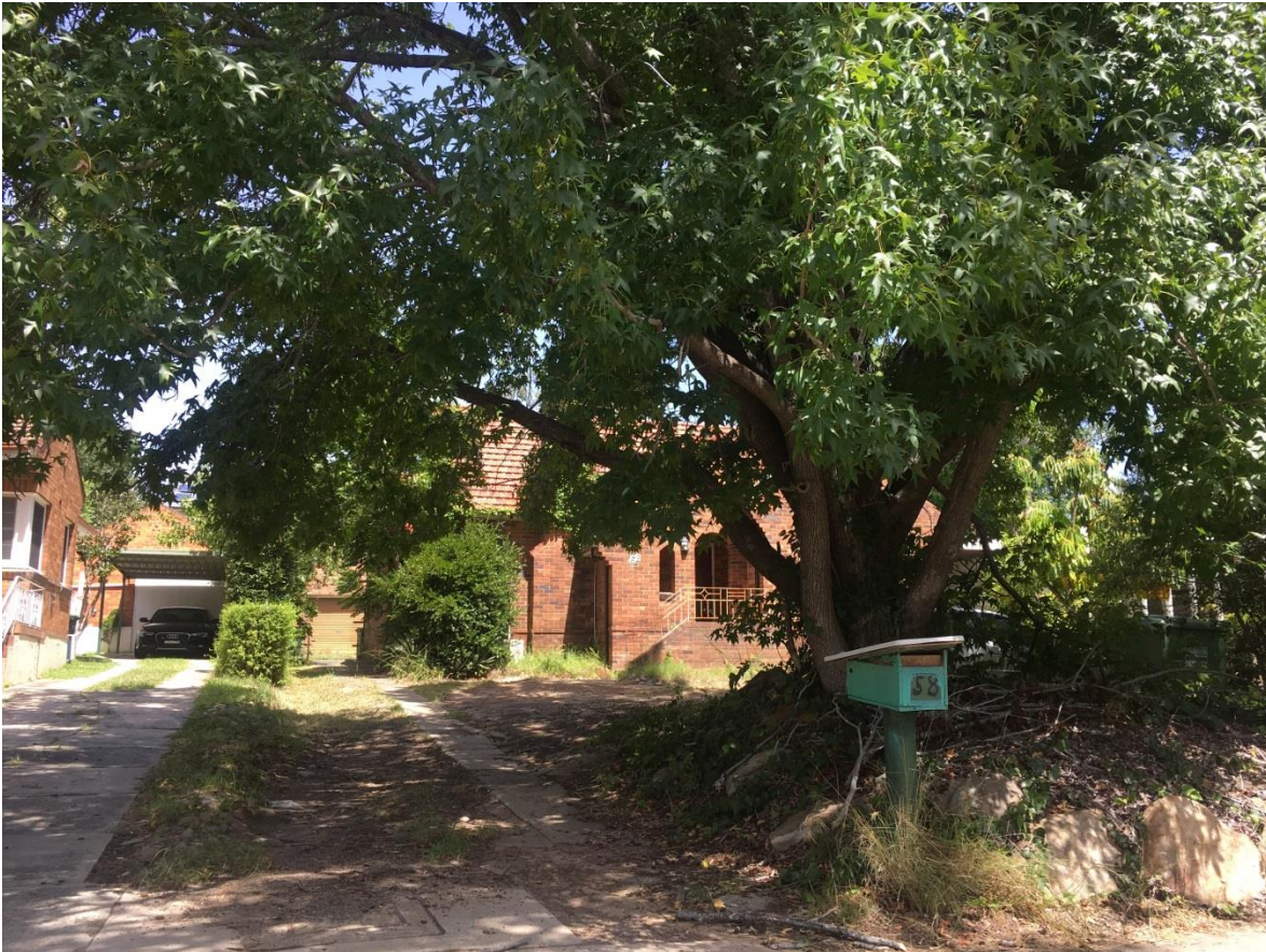
Figure 8: Front elevation of the existing dwelling house at 58 Beresford Road
