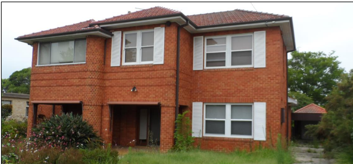
Figure 3: Front façade of the subject site at 12-14 Elwin Street, Strathfield.
