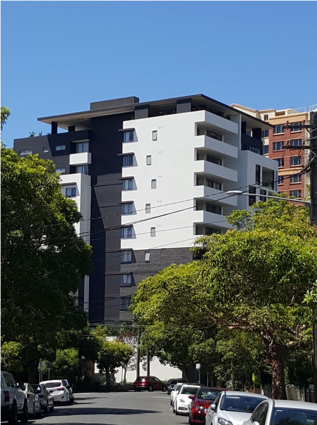
Figure 3: North easterly view of the subject building from Churchill Avenue
