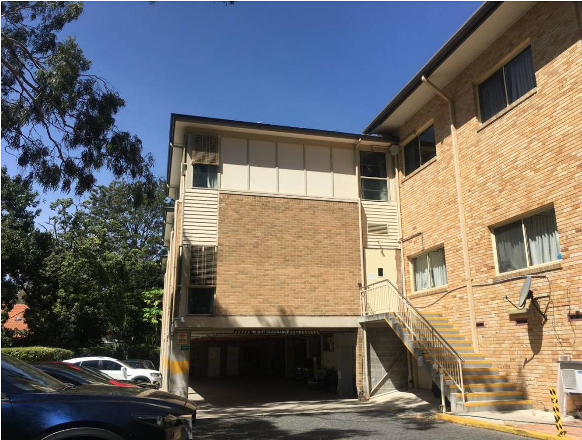
Figure 6: Rearmost portion of the existing residential care facility, including car parking area (and undercroft parking area)
