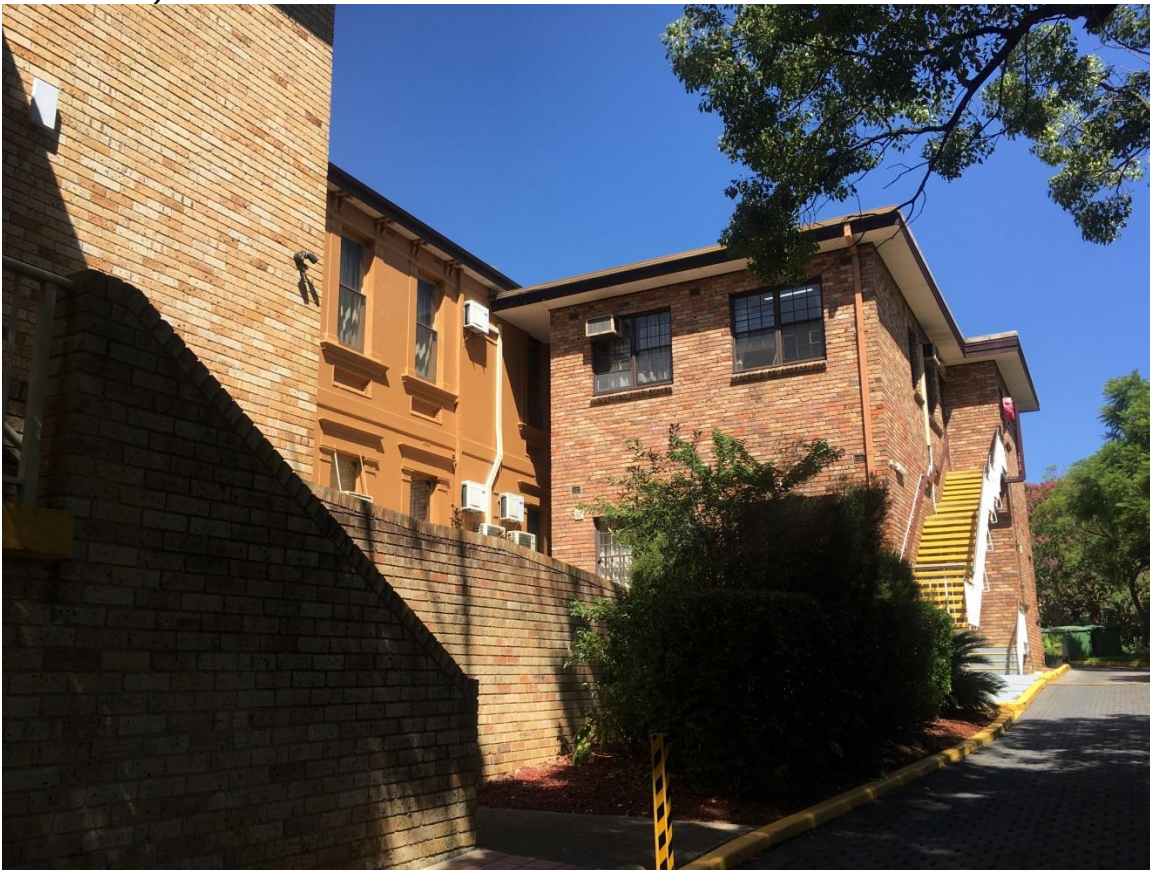
Figure 5: Portion of the south- western side elevation of the existing residential care facility
