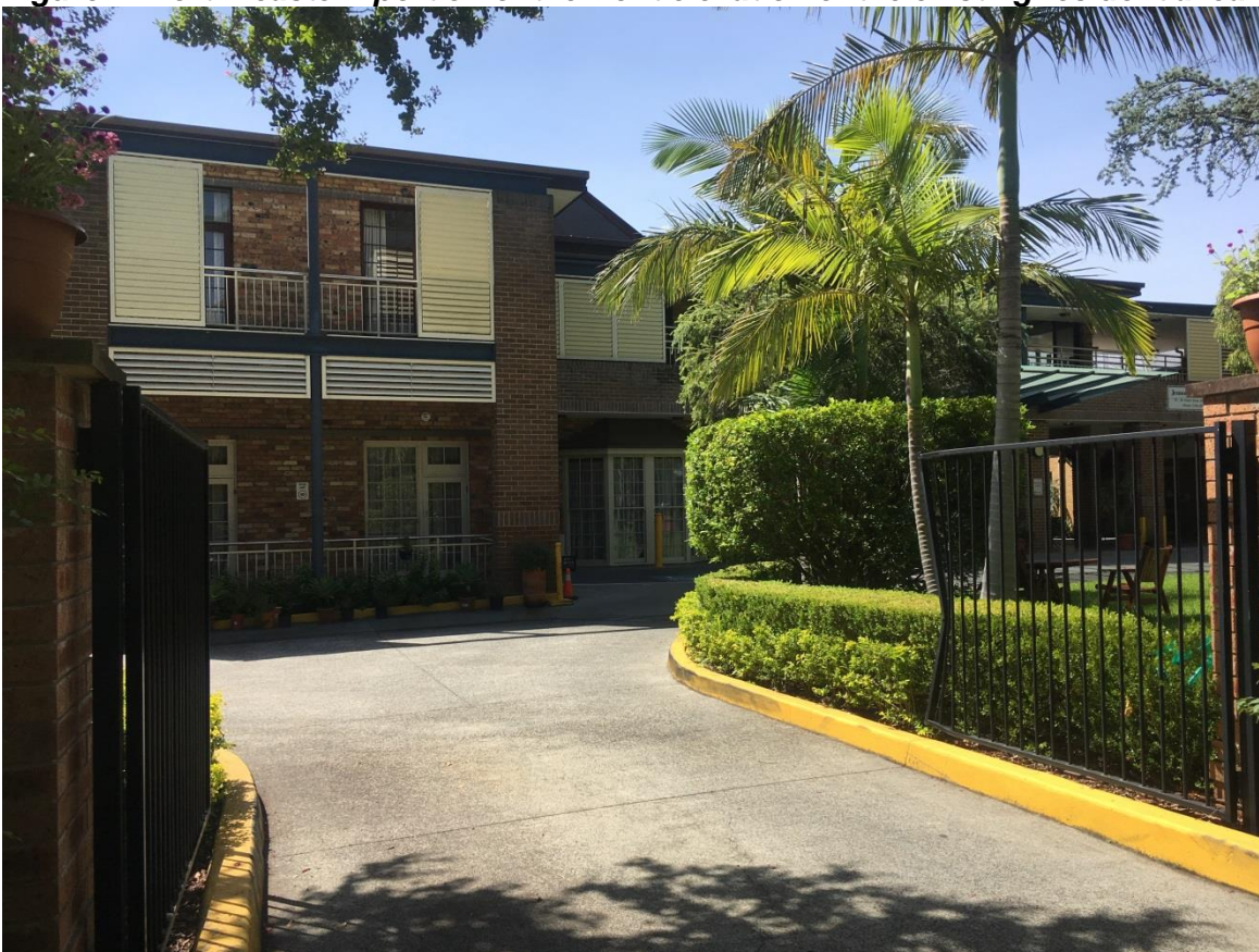
Figure 3: South- western portion of the front elevation of the existing residential care facility
